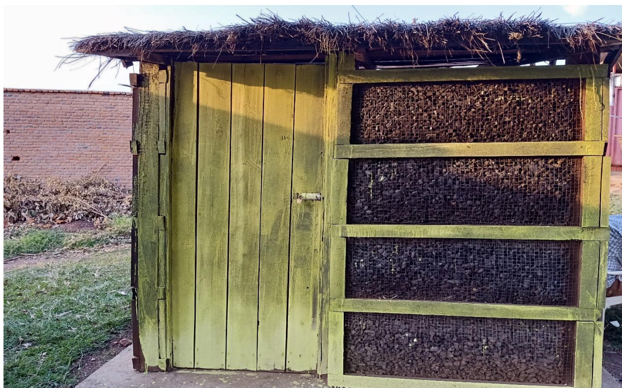
Figure 8: Charcoal coolers constructed by ABIN in Bubanza
